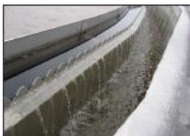
Betonrende med: KD 16.17 Flydeslamskant. KD 16.14 Hakkant.
