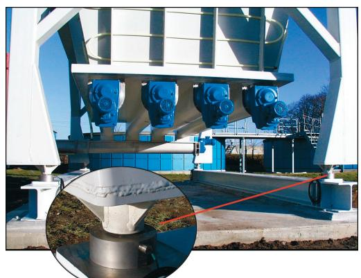
The outlet is collected in a sectional screw KD 02. From this point the sewage can be further conveyed by means of shaft less screws KD 02. On the rounded picture is shown a load cell, assuring a constant control of the level of sewage in the silo.
