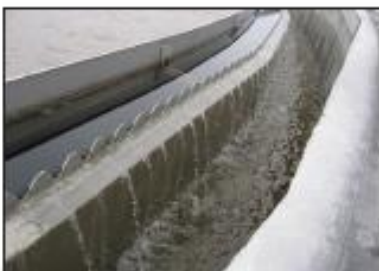
Betonrende med: KD 16.17 Flydeslamskant. KD 16.14 Hakkant.
